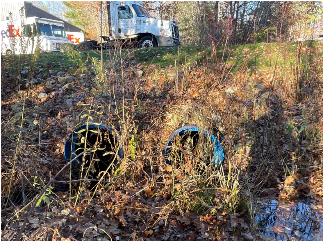
Stream S-KMN-2, culvert inlet on northeast boundary of Survey Area November 2, 2022.
