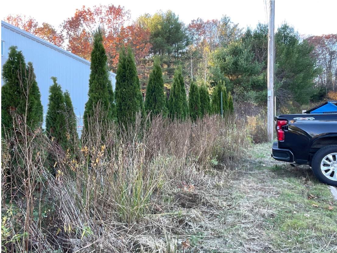
Upland Drainage adjacent to parking area November 2, 2022.
